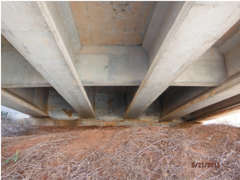
Underside of Bridge at End Bent
