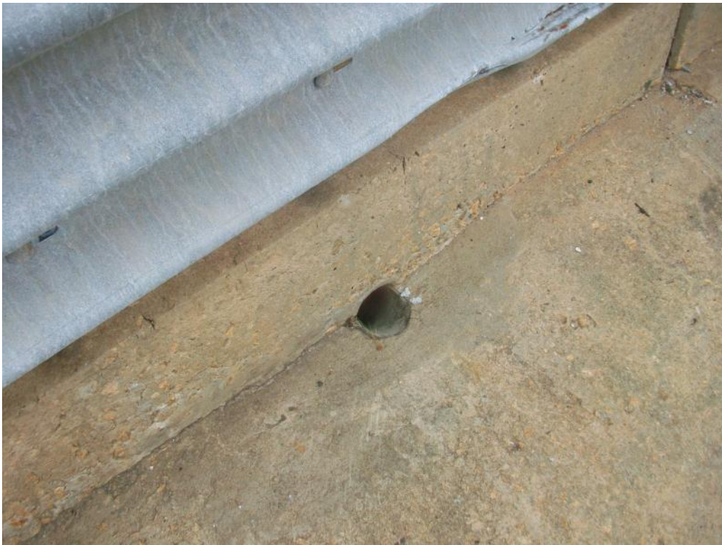
Photograph 3 – Typical view of asbestos containing transite drain pipe located on the bridge structure.
