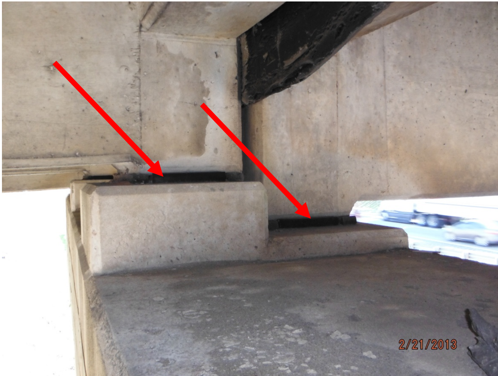
Asbestos-Containing Interior Bent Cap Pad
