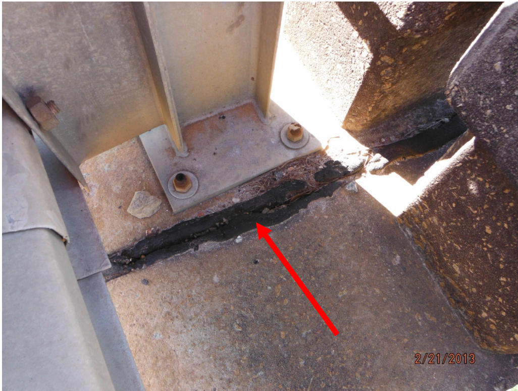
Asbestos-Containing Expansion Joint Material
