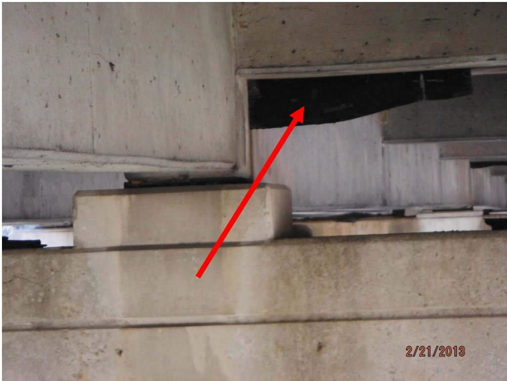
Asbestos-Containing Expansion Joint Material
