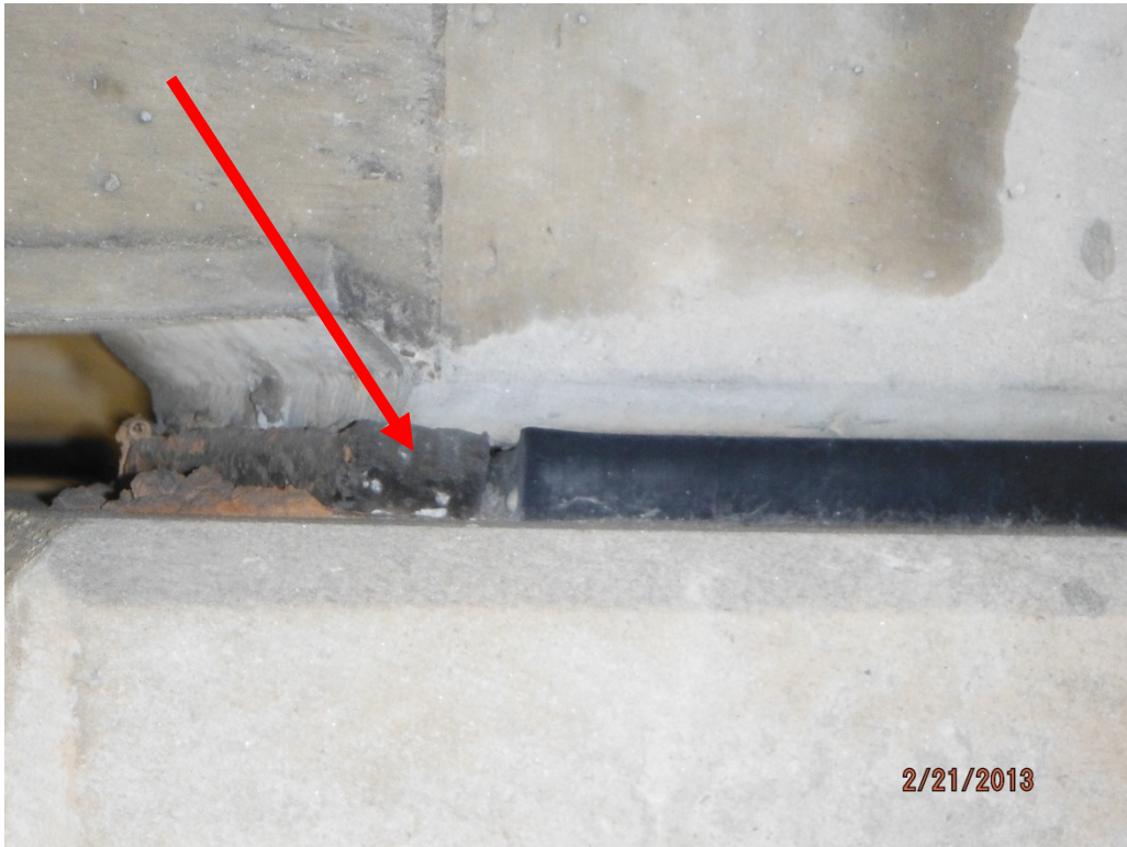
Asbestos-Containing Interior Bent Cap Pad
